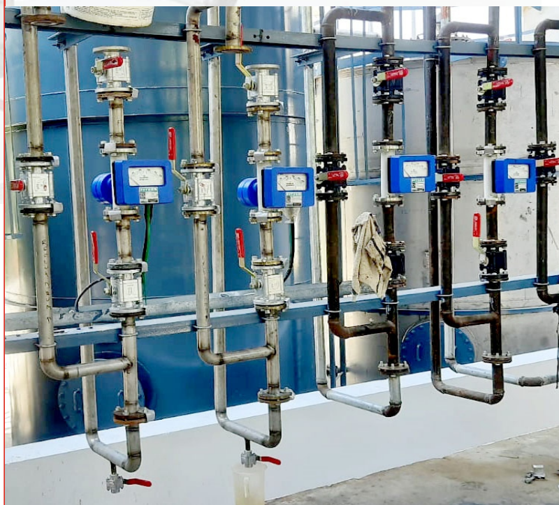
INSTALLED ROTAMETERS IN PLANT
